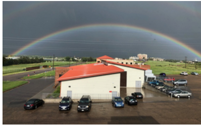
Advanced Beam Laboratory (ABL)
